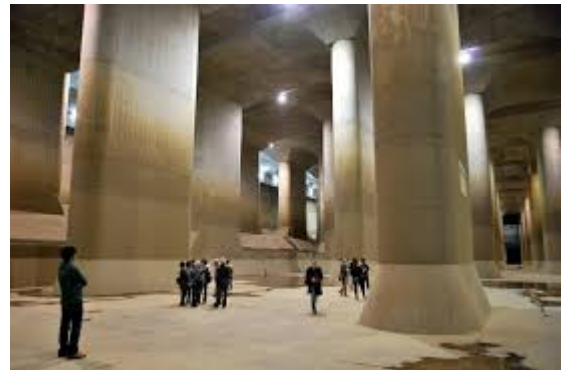
Fig 5 Underground discharge channel – (Source: Neeraj.S, Manekar and Shritej A Nirmal 2015 on Advanced Drainage System Tokyo, Japan.)
